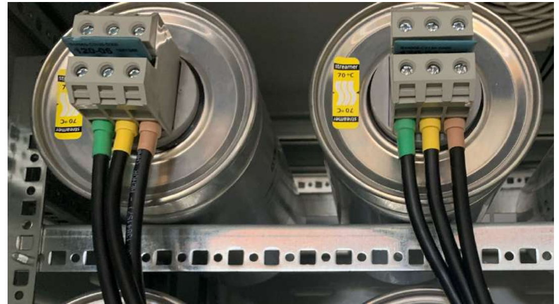
Installation of vFPTs on the capacitors
